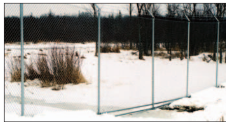
Shown above is a finished portion of the 27,000-lineal-foot job. The 10-foot-high fabric was installed on SS40 framework. The height was necessary to help prevent deer intrusion onto the runways, a constant and potentially dangerous problem. At right, Delta's trusty Ford tractor makes deep tire prints in the snow, although at times the snow was much deeper. While the crew avoided the worst snowfall, which came after the job was completed, cold and rain were the big enemies.
