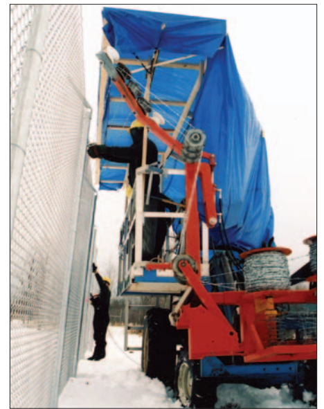
Shown above is a finished portion of the 27,000-lineal-foot job. The 10-foot-high fabric was installed on SS40 framework. The height was necessary to help prevent deer intrusion onto the runways, a constant and potentially dangerous problem. At right, Delta's trusty Ford tractor makes deep tire prints in the snow, although at times the snow was much deeper. While the crew avoided the worst snowfall, which came after the job was completed, cold and rain were the big enemies.
