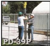
The **PD-39P Panel Post Driver** ensures fast erection of temporary panel fencing. It is easily operated by one worker.
